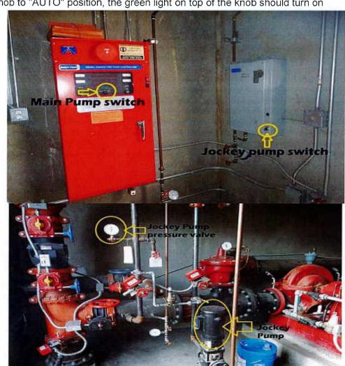
the knob to "AUTO" position, the green light on top of the knob should turn on
